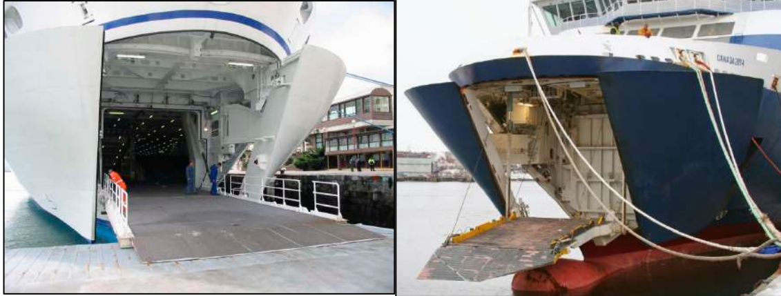
Watertight doors on a ferry
