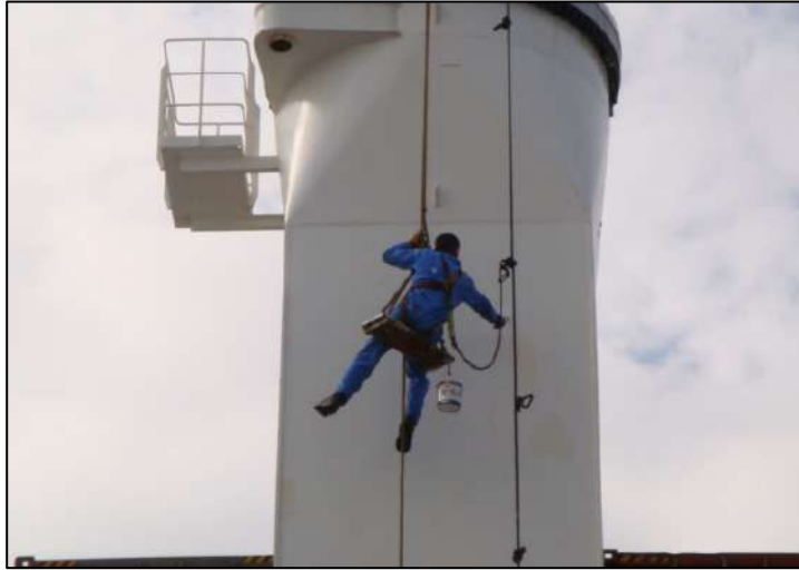
Safety harness attached to safety line and tools/paints secured against falling
