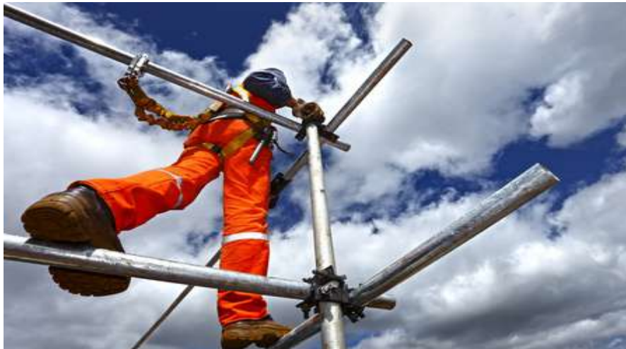
Figure 39 – Correctly erected scaffolding
