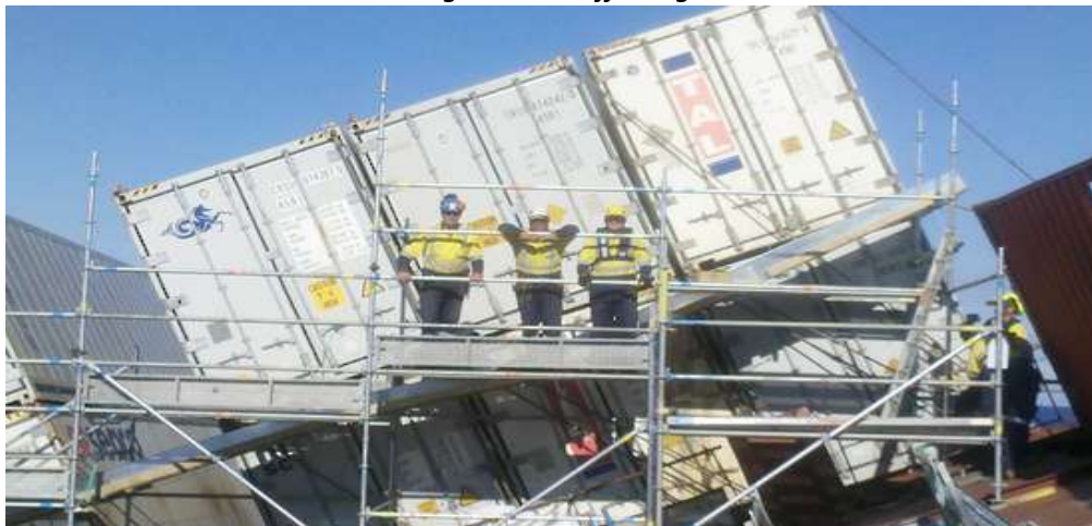
Figure 42 Scaffolding erected on board a ship that is listing to port
